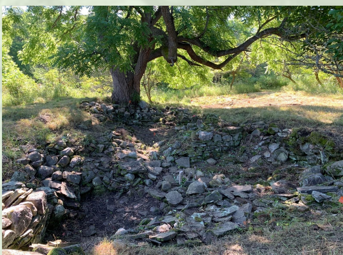
Image 3: The visible remains of the dry-stone foundation of the Hall Residence, with the eastern sections towards the front and the western section in the back next to the tree.
